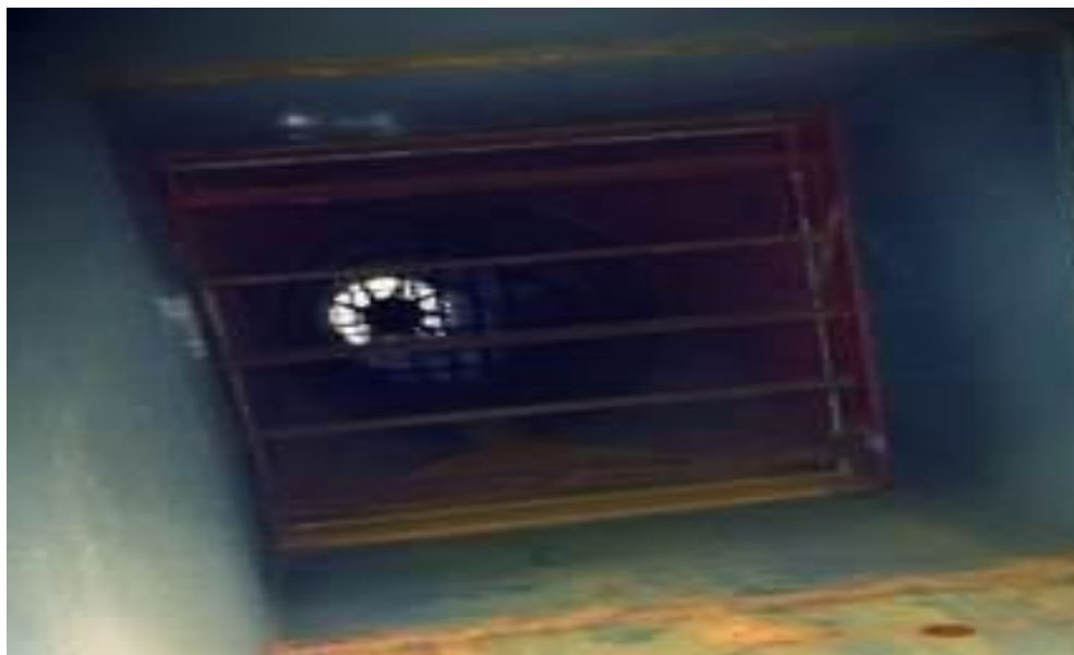
Figure 6.7. Louver blades at 0° angle position
